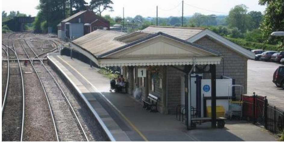
Castle Cary accessible footbridge
