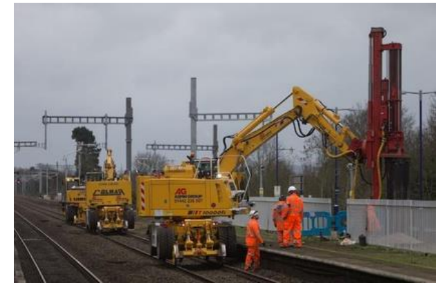
Great Western Electrification
