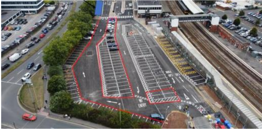
Gloucester station forecourt improvements
